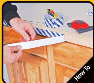
Remove liner, apply edgebanding
